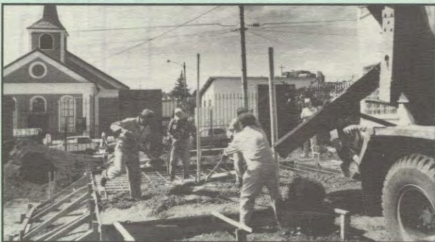
Pouring the concrete for the ALAS satellite antenna at HCJB.
