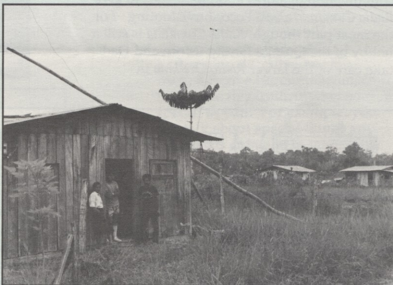
Señora Quinga, son Marco and Angel at the Radio Cumandá transmitter building
