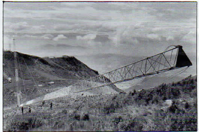
Raising the new tower (the old tower is to the far left of the picture). Quito city can be seen in the valley.
