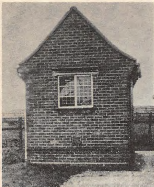
Coaxial repeater station
