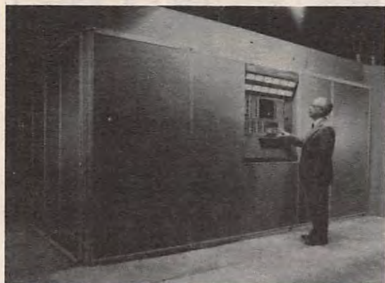
Final testing of completed transmitter
