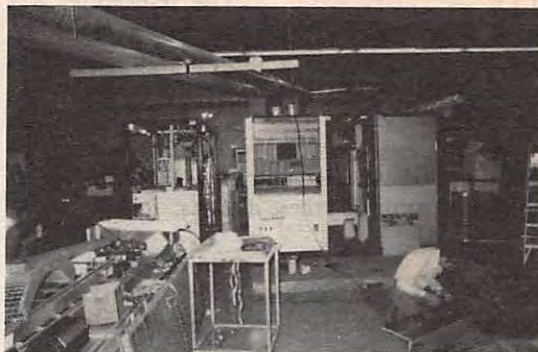
Transmitter tear down begins
