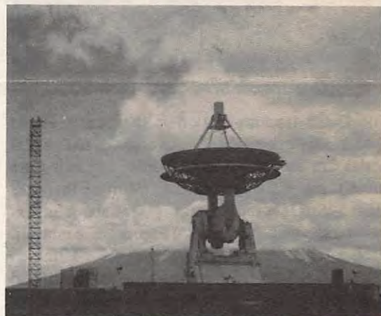
12-meter dish antenna
