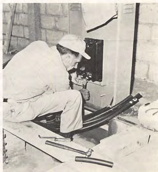
Stan Houghton makes final connections
