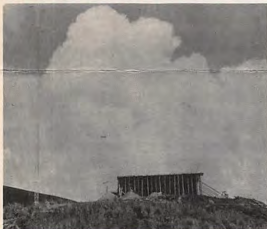
Construction on mountain top
