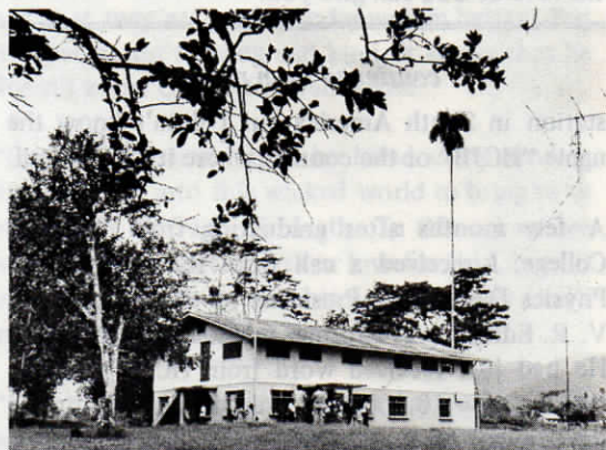
HCGM-7 Studio-Transmitter Building
