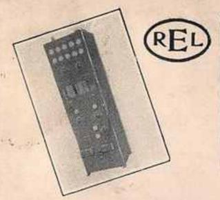
W2XV 100 watt crystal control transmitter 4795 kilocycles 62.5 meters. Zeppelin half wave voltage feed antenna.
